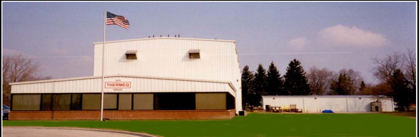
Front with view of offices, high bay facility, and back facility.
