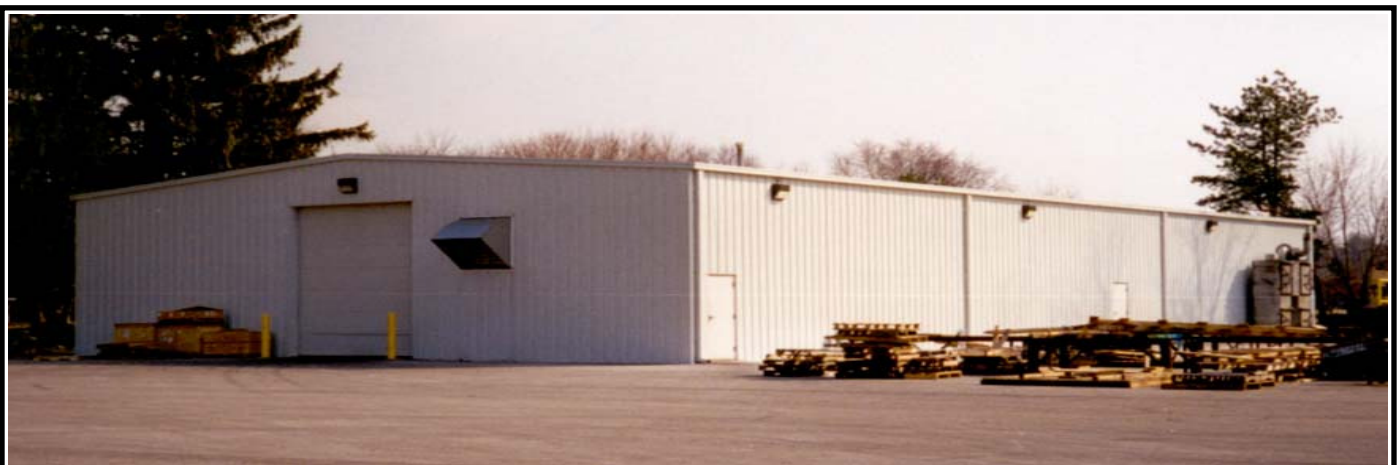
Back facility which is divided into cells for standardized component manufacturing.
