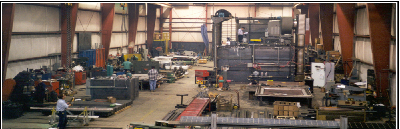
High bay facility utilizes two cranes for fabrication, assembly, and shop testing.
